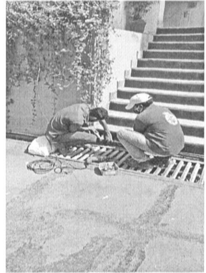
Electricians: Maintenance of Cables.
