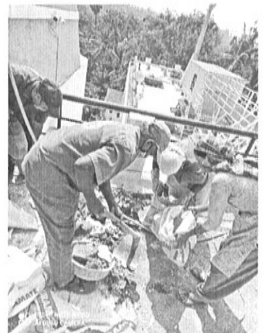
Masons: Pre Monsoon Water proofing at Rahaman College terrace.
