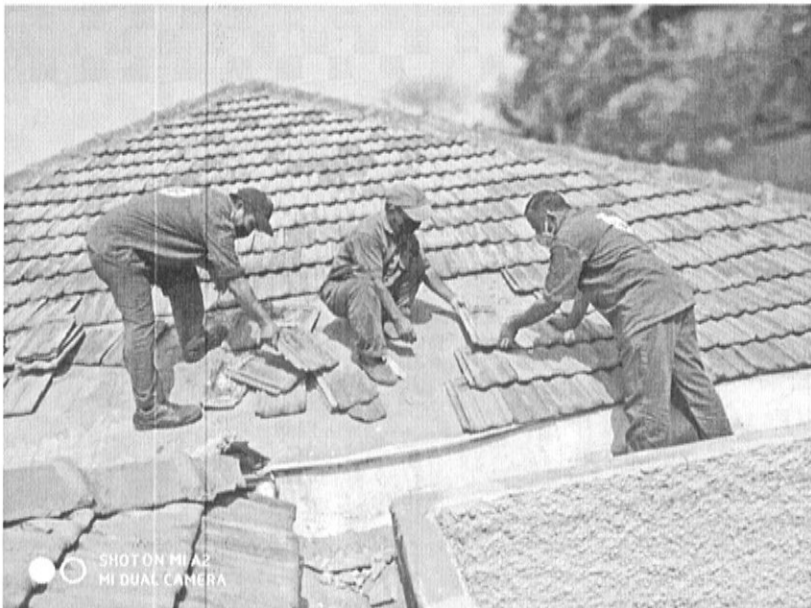
Carpenters: Pre Monsoon water proofing at Barnes Academy.
