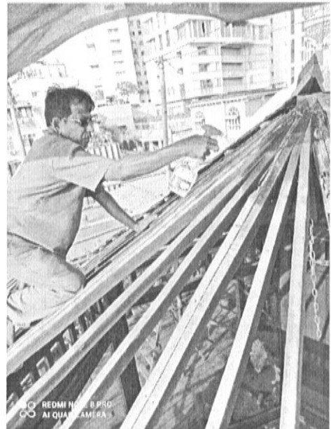
Carpenters and Polishers: Wooden Roof repairs of Chairmans Bungalow at Worli
