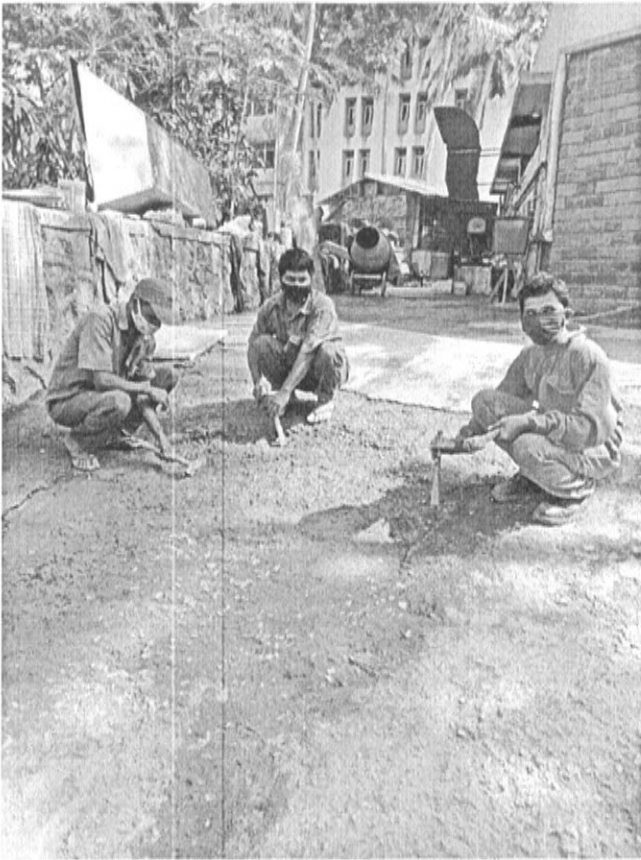
Painters: Pre Monsoon water proofing at GC Library.
