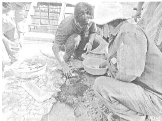
Masons: Pre Monsoon Water proofing at Rahaman College terrace
