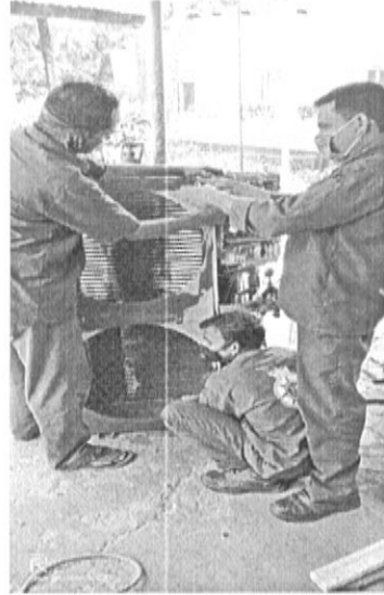
Welder and AC Mechanics: Body repairing of AC's of Worli. Welder and AC Mechanics.
