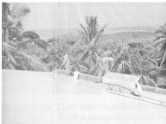
Painters: Pre Monsoon Water proofing work at Shangrila Building terrace
