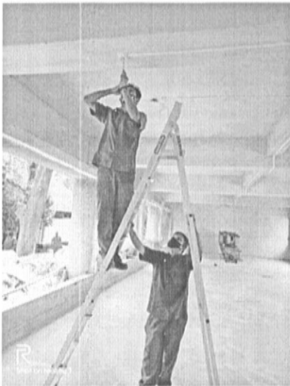
Wiring of New training workshop: Electrician.
