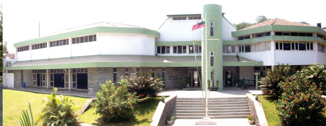
Administrative Office & Dining Hall
